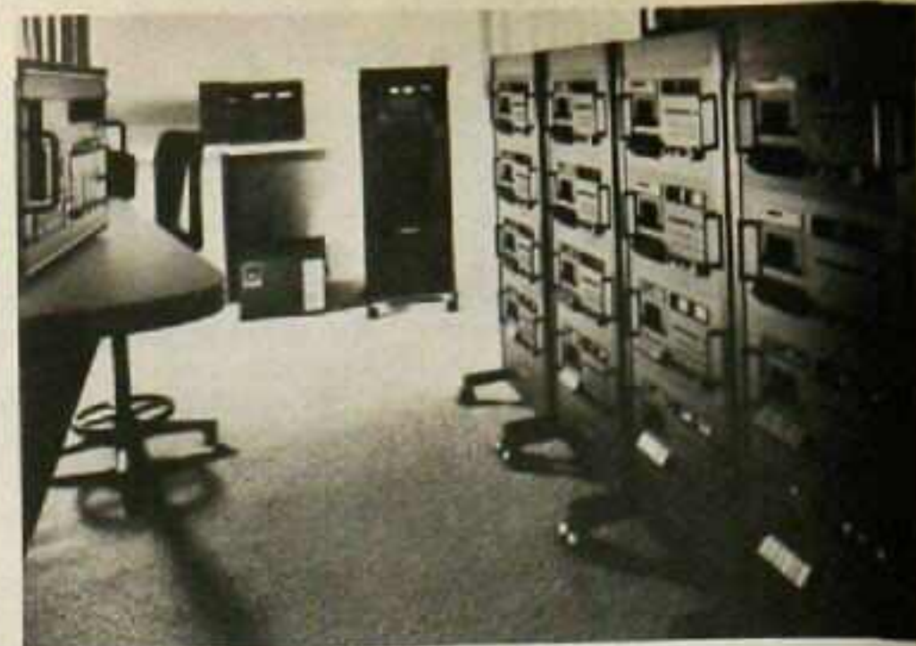
Taping room real-time cassette duplication facility uses 16 rack-mounted Nakamichi series 600 cassette consoles.
