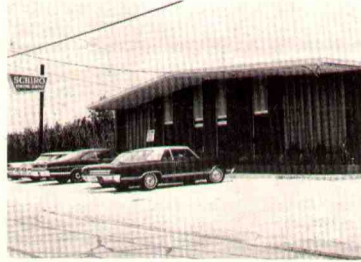
NEW SCHIRO VENDING SUPPLY building in suburban Metairie has over 10,000 square feet.
