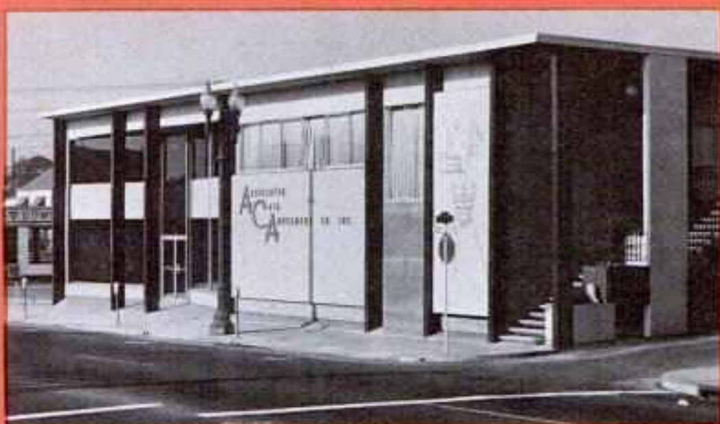
ACA Headquarters, Oakland, California
