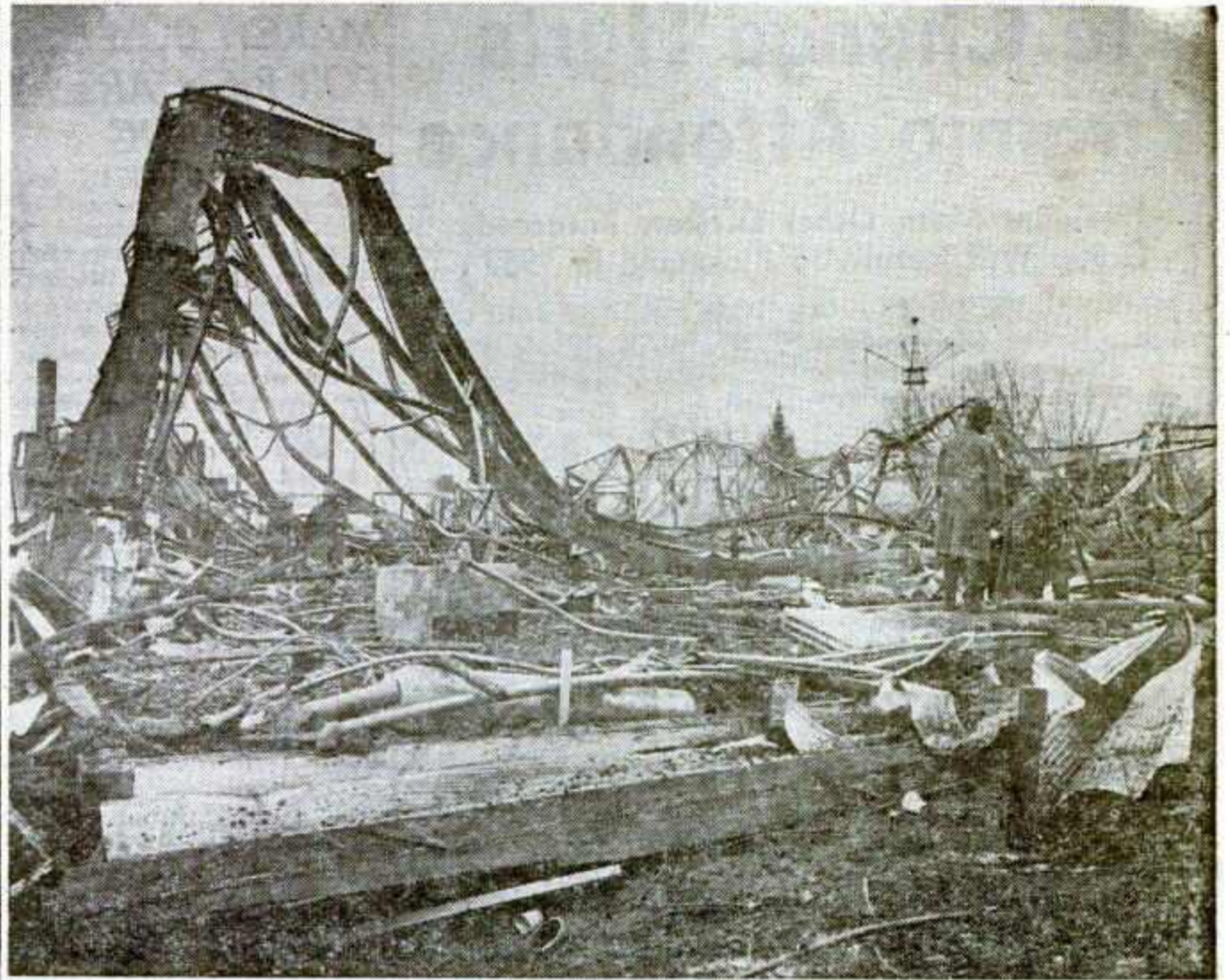
TWISTED GIRDERS ARE ALL THAT REMAIN of Iceland, the venerable ice rink at Carlin's Park, Baltimore, which burned to a skeleton last week. The seven-hour blaze was difficult to combat due to ammonia fumes originating in the refrigeration system, and cause of the fire has not been determined yet. A Baltimore Clippers professional hockey game had been played the previous night. Identifiable objects are the park's airplane swing tower in the background at right and a charred Coca-Cola box, center. President William J. Fischer said the $175,000 loss was covered by insurance, which is enough to build another rink.
