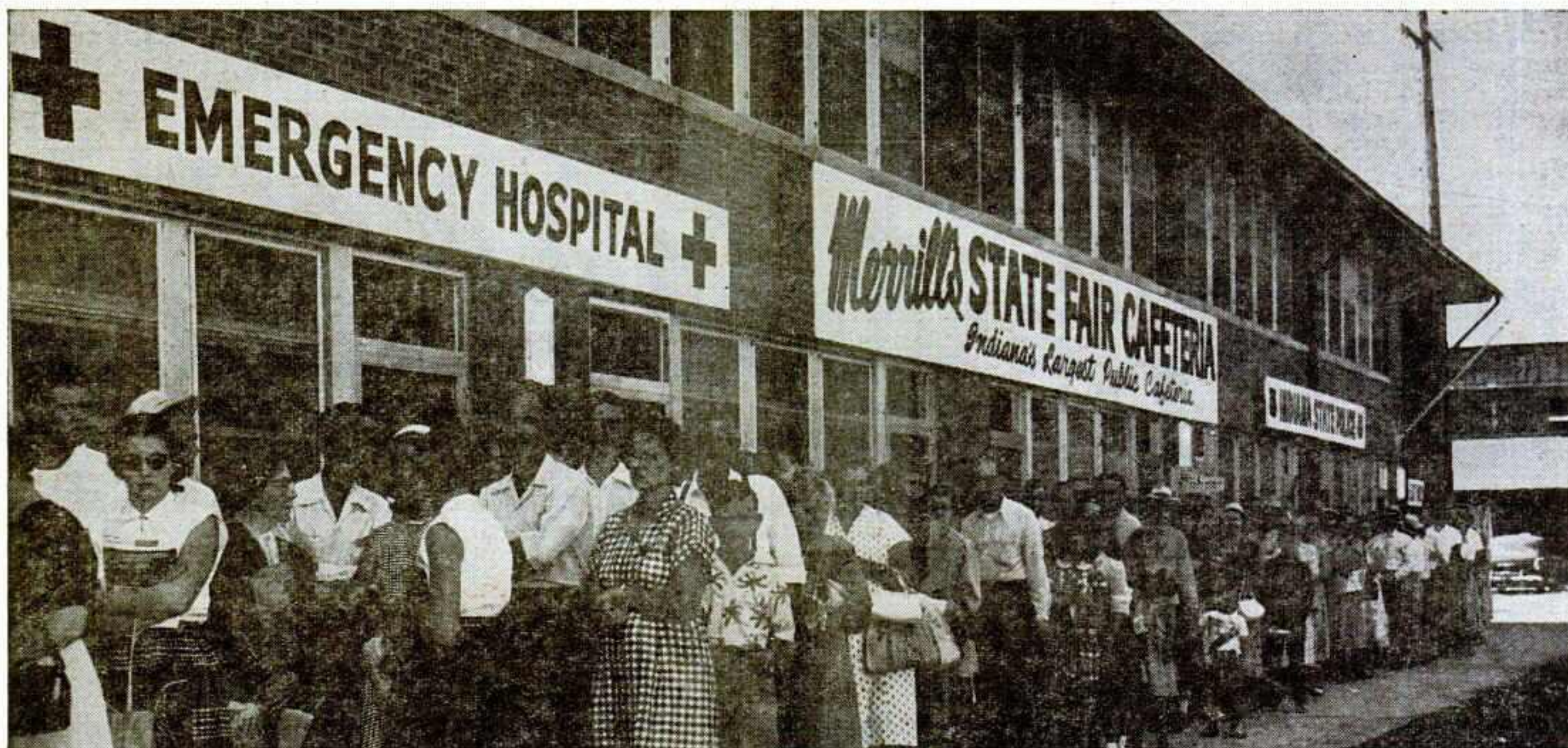
The Indiana State Fair's new $300,000 Service Building not only serves to centralize functions of many of the annual's utilities but proves a popular eating place for thousands of patrons. The long waiting line attests to the quick acceptance accorded the unique cafeteria which operated on a pay-before-you-eat basis. The Red Cross emergency hospital and the Indiana State Police quarters, two of the service units in the center, are also shown.
