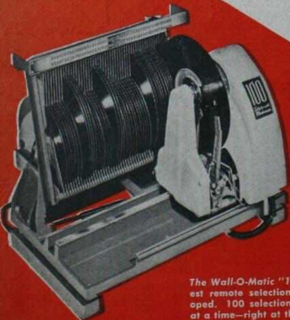
The Select-O-Matic "100" Mechanism. Plays 10 and 12-inch records without presetting. By any comparison, the most revolutionary development in the history of the coin-operated music industry.
