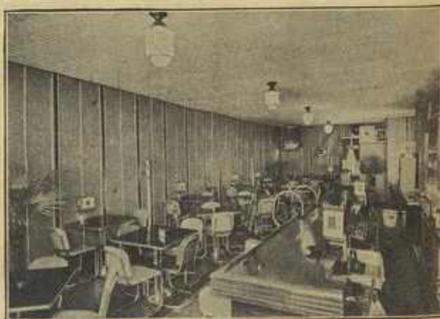
KEENEY WALL BOX REMOTE-CONTROL EQUIPMENT is featured in the Dull and Bruner Wonder Bar, Fremont, O. The Findlay Music Company, Findlay, O., made the installation, and reports gains in revenue since the Keeney equipment was installed.
