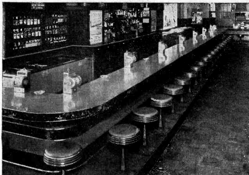
INSTALLATION IN COTTON CLUB, Indianapolis, of Pla-Mor remote-control equipment made by the Packard Manufacturing Company. The installation was made by the Central Distributing Company, Indianapolis.
