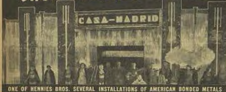
ONE OF HENNIES BROS. SEVERAL INSTALLATIONS OF AMERICAN BONDED METALS
