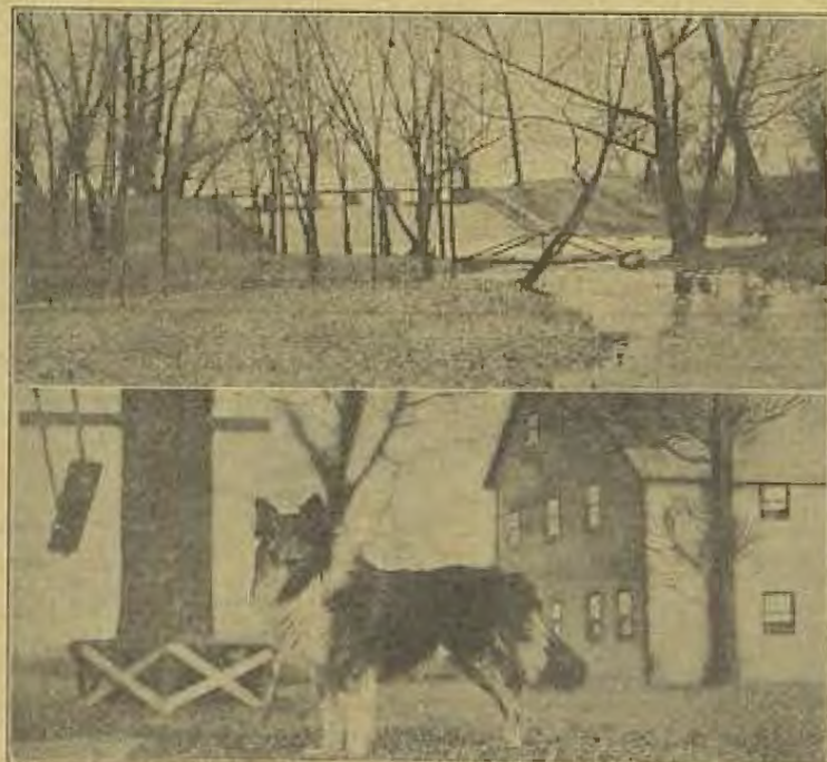
THESE TWO VIEWS EXAMPLE PROGRESS AND STABILITY: Top picture shows the power dam of the Hydro-electric plant which furnishes light and power for the winter quarters of the Northeastern Shows of which F. L. Flock is the executive head. The power plant is owned by the shows and is located in the Detroit, Mich., sector. In the shot below can be seen the quarters building and in the foreground is Rex, educated canine, who is the official watchman for the entire properties and may be seen in the top picture making his rounds.
