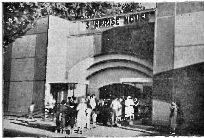
IN EUCLID BEACH PARK, Cleveland, where President Harvey J. Humphrey is anticipating one of the biggest seasons in many years, the Surprise House, modern front of which is shown here, is one of the innovations. It is replete with astounding effects which are worked thru radio control and without use of visible mechanism or the electric eye.
