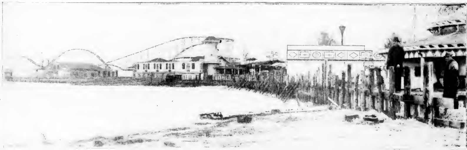
Pleasure Beach Island, famed as the hiding place of some of Captain Kidd's gold, was being slowly washed away. Half a mile of bulkheading, which also will be utilized as a new auto shore drive, was required to stop the Sound's encroachment. Pleasure Beach Park is undergoing steady improvement under the able direction of Fred W. Pearce, general manager, and is becoming one of the leading amusement resorts of New England.
