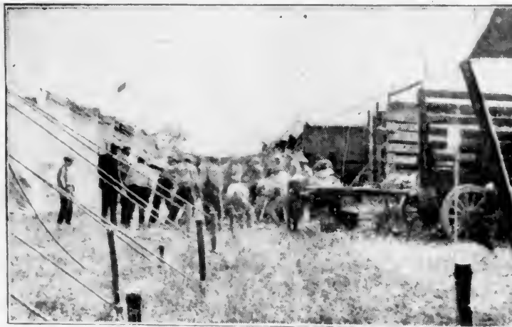
When dark, ominous-appearing clouds overspread the sky after the big top is up experienced circus men keep a weather eye out for a big blow. In the accompanying picture a gang of men is shown "guying off" to protect the tents from a bad wind. Sparks' Circus at Woonsocket, R. I.
