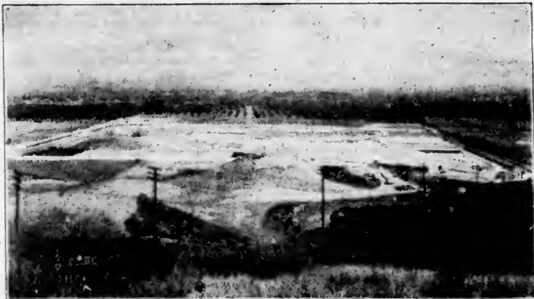
The tent shown in the accompanying view of the Pomona (Calif.) fair grounds attracted many people to the fair by reason of its size, many people going all the way from Los Angeles just to see the tent. It was an eleven-pole top, 130 feet wide by 550 feet long, and was put up by Tom Kennedy, well-known Western canvasman. The tent is the property of the National Orange Association, of San Bernardino, and was made by the Baker & Lookwood Co., Kansas City.
