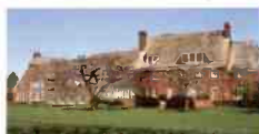
SOUTHAMPTON, NY Architectural Masterpiece: Estate sections $22,000,000. WEB: BB0054203. Southampton Brokerage, Harold Grant, 631.283.0600 Ext. 13
