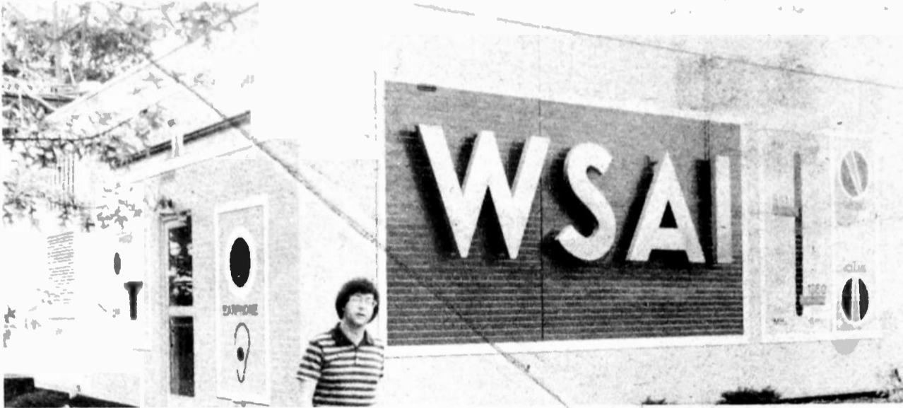
CINCINNATI'S BIGGEST RADIO —Assistant PD Ted McAllister walks past WSAI's transmitter building which is designed as a giant radio.
