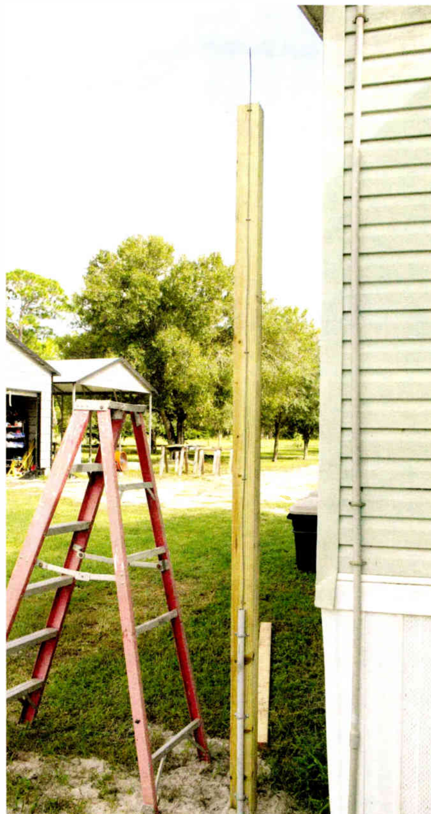
Fig. 1: The down conductor has been stapled to the 4-by-4 pole.
