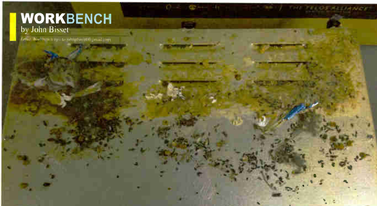
Fig. 1: DA parameters out? No, the antenna monitor was being used as a mouse outhouse. The top vents on the monitor served to channel liquid inside, destroying printed circuit boards.
