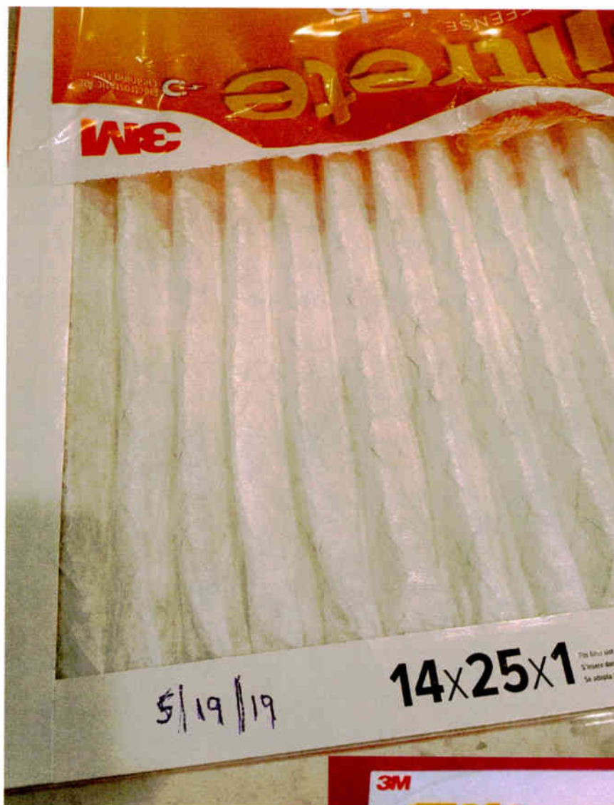
Fig. 1 (above): Don’t forget air handler filters — and make a notation when the filter was changed.
