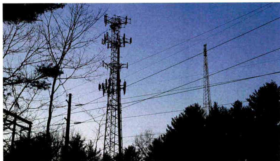
Fig. 2: AM engineers need to keep an eye out for new tower construction. Cell towers can seem to appear overnight!
