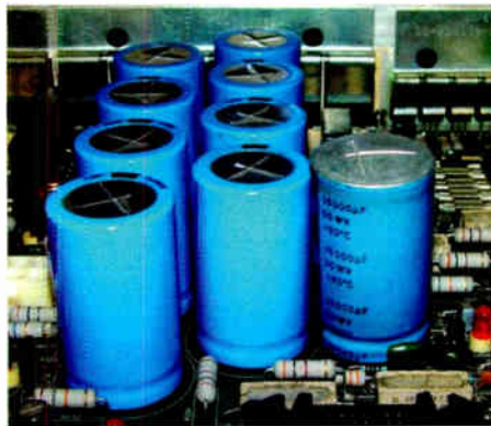
Fig. 3: The capacitor bank after replacement, with a "bad" capacitor on the right.
