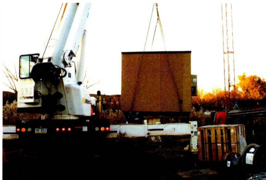
Fig. 2: One of four Thermobond pre-cast concrete building is being off-loaded.
