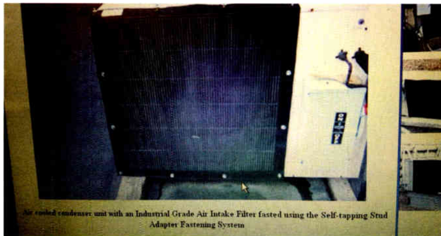
Fig. 3: An example of the installed mesh filter from Air Solution Co.
