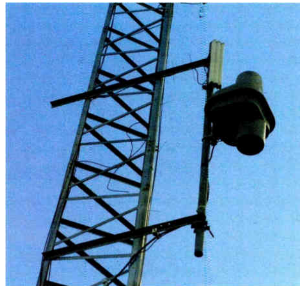
Fig. 1: A good reason to view your FM antenna periodically with a pair of binoculars. The unexpected tenant is visible above the Shively bay.
