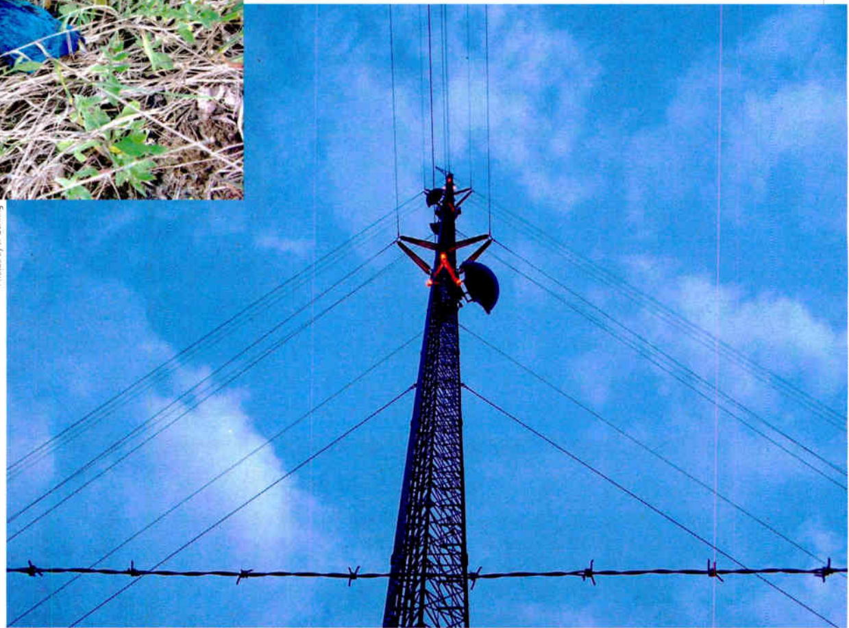
Non-flashing (i.e., steady-burning), L-810, tower lights attract migrating birds and can cause them to collide with tower guy wires and the tower structure.
