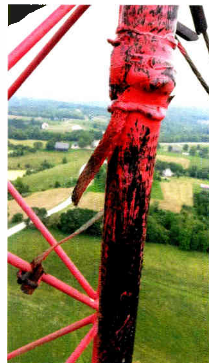
Fig. 2: Your climber might also spot a broken ground kit.
