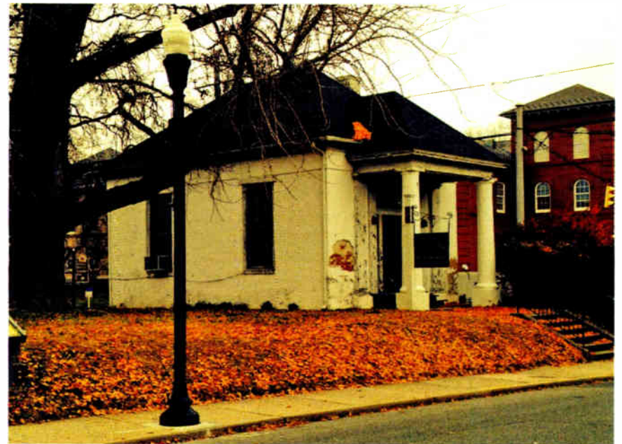
The Wallace Office building, a Civil War office used by Col. James W. Wallace for enlisting local troops and militia, is under restoration and will not be available for use in time for WHCP sign-on. Note the Cambridge Courthouse in the rear.
