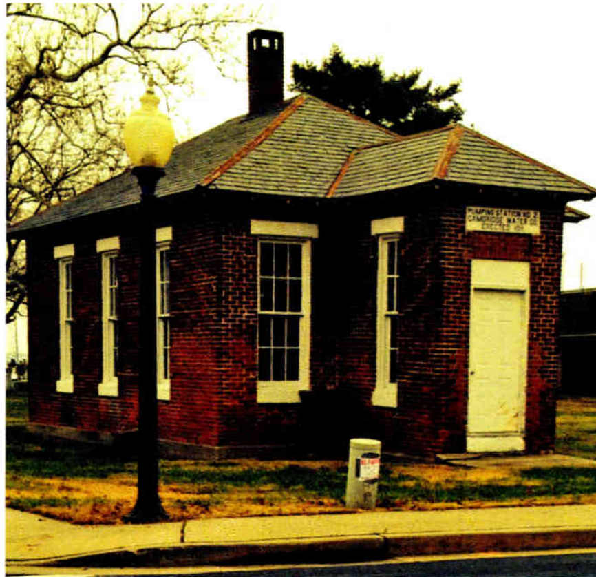
The vacant water pumping station by the Cambridge Marina frequently floods.
