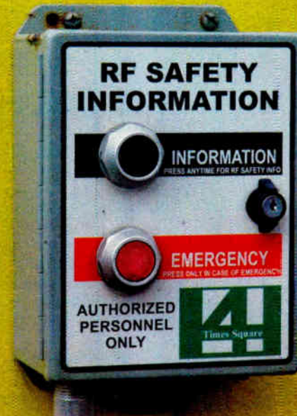
The Durst Organization recorded RF safety information at 4 Times Square in New York for those who need access to the rooftop transmission site.
