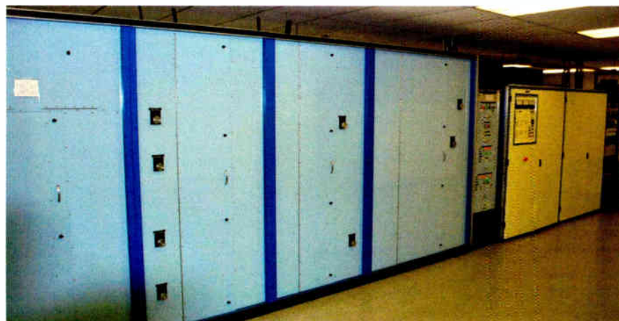
KMZT(AM) recently invested in new equipment including Nautel transmitters (a 25 kW main and 12.5 kW aux) as well as a Kintronic Labs phasor. Writes author Saul Levine, 'We put our money where are convictions are for AM.'
