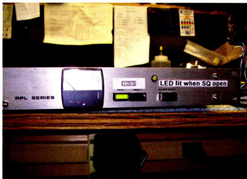
The front panel showing the completed modification.
