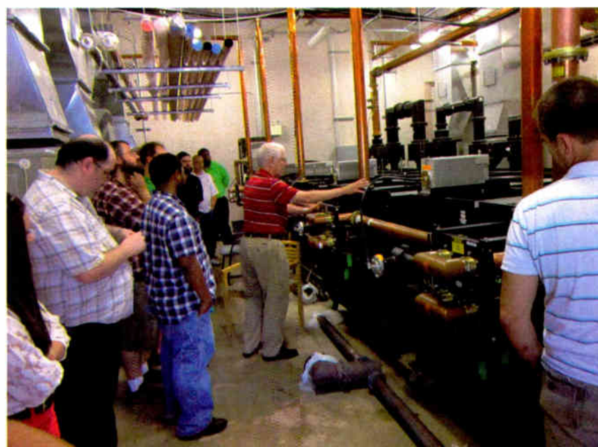
Frank Giardina discusses FM combiner operation at a multi-station transmitter plant.
