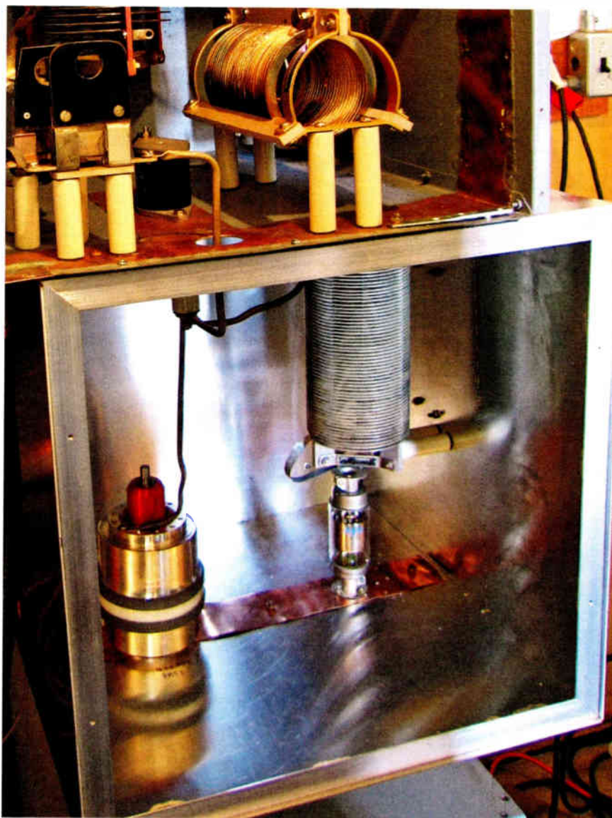
The station hired Kintronic Labs to design a filter to nudge WJON into compliance with FCC rules.
