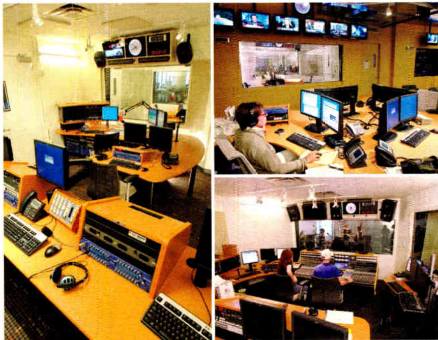
New York Public Radio's facility will be featured. Shown, clockwise from left: Control Room 2; the News Hub, where elements of newscasts for WNYC(AM/FM) and WQXR(FM) are created; and Control Room 5, where WNYC(FM)'s music show "Soundcheck" is produced. The API Vision console has a custom insert to interface with an SAS 32KD router system without using an outboard mixer.
