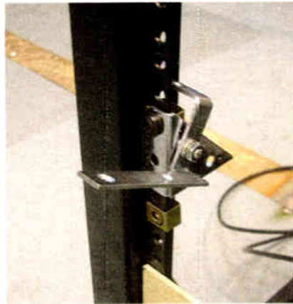
Fig 2: The combination of bolts, nuts and 'L' and angle brackets will be used to secure the rack panels.
