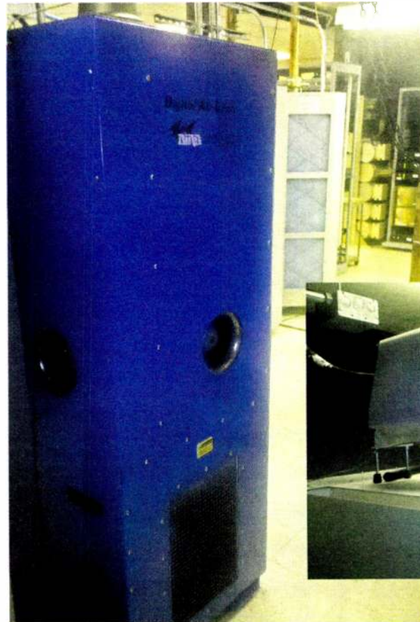
Left: Air-cooled dummy loads like this 20 kW unit grace medium-powered radio stations throughout the world; no water for cooling is required.
