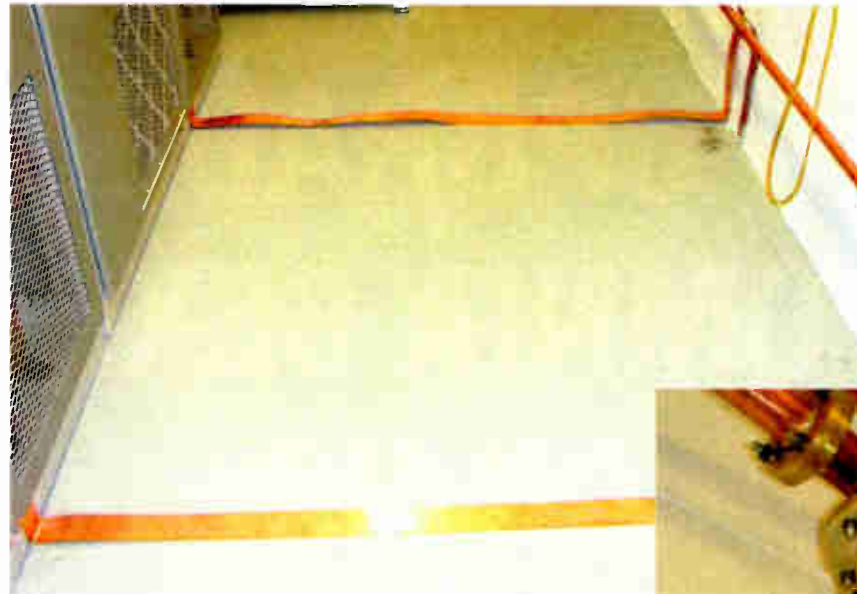
Fig. 1: Proper transmitter grounding. Make sure the ground strap is connected to ground.
