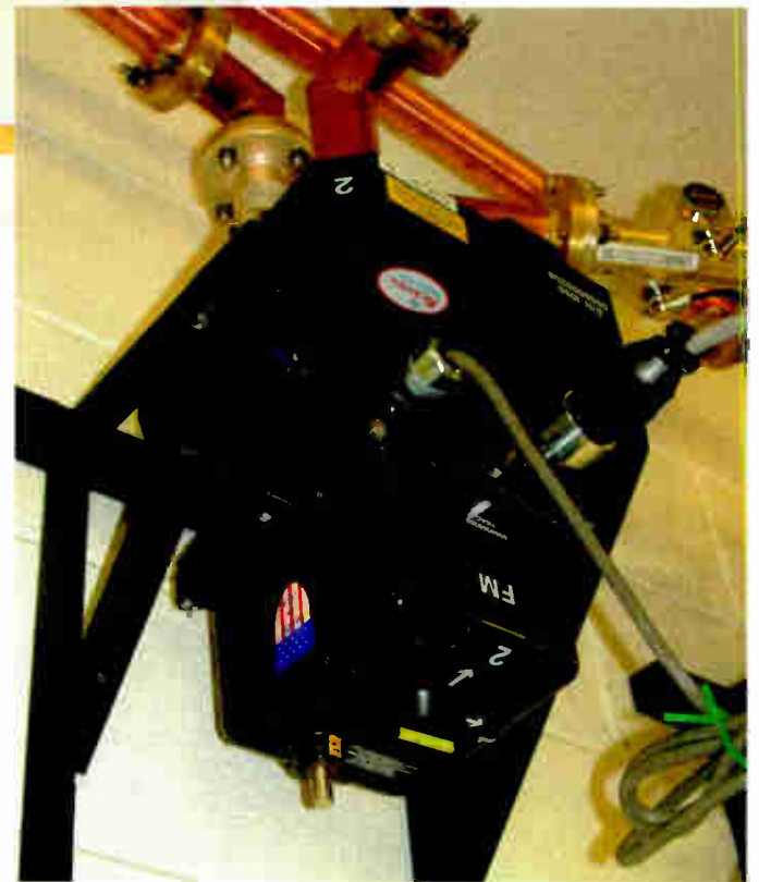
Fig. 2: Buy a pre-wired RF switch connection cable to ensure that control and interlocks are connected properly.
