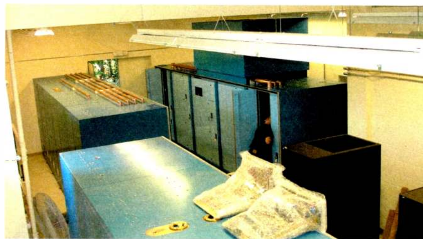
The three phasors are placed in the building and assembled.
