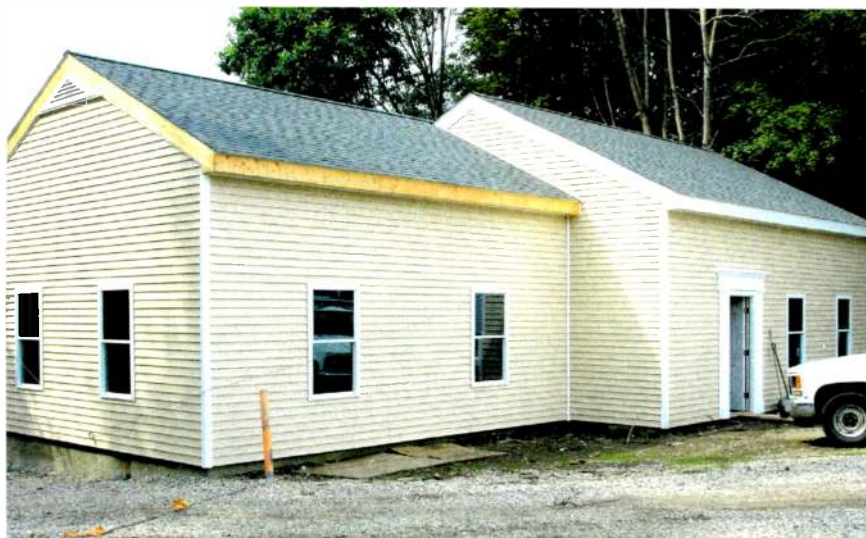
The original WUNR transmitter building had a flat roof. Clear Channel had to make the building look like surrounding houses. The windows are fakes.
