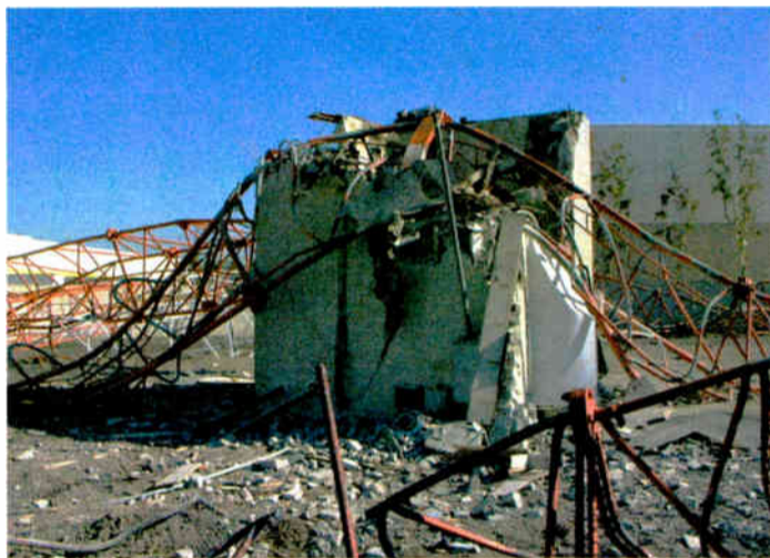
The KFI tower and destroyed antenna tuning house as they looked after the tower collapsed, having been struck by a small aircraft in 2004.
