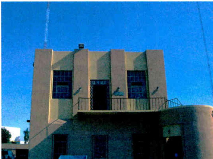
The KFI transmitter building in La Mirada. The replacement tower can be seen on the left; on the right is visible the 200 foot aux tower, which had been in use at 25 kW since the main was knocked down in 2004.
