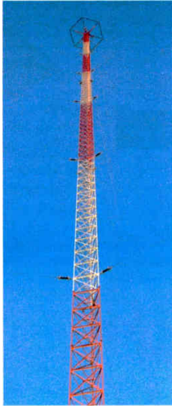
A view of the KFI tower, standing 684 feet AGL, with its top hat. The Clear Channel station airs at 640 kHz.
