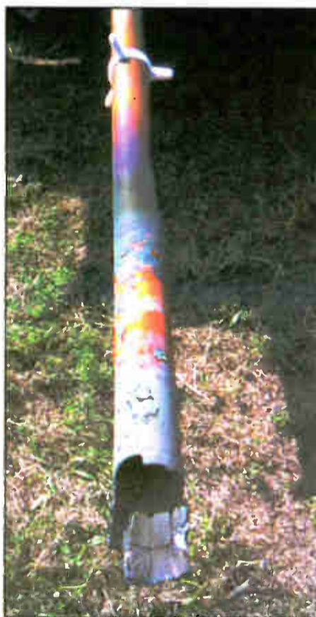
Fig. 2: The real damage occurred some 70 feet below the top bay. This inter-bay line was melted by the sustained RF arc.
