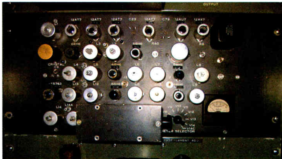
About one-third of the resistors and capacitors had to be replaced in the exciter.
