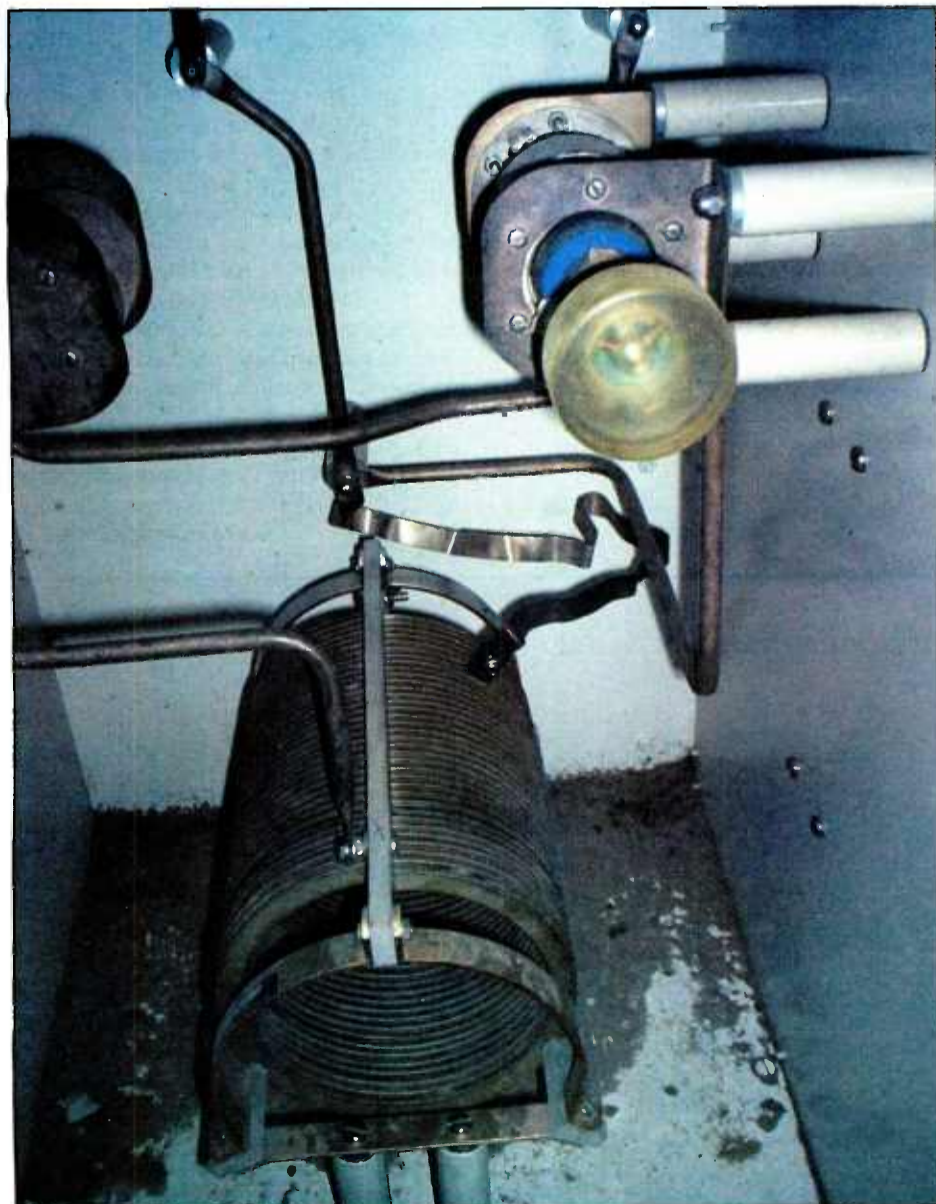
Fig. 3: View of coil assembly after being repaired.
