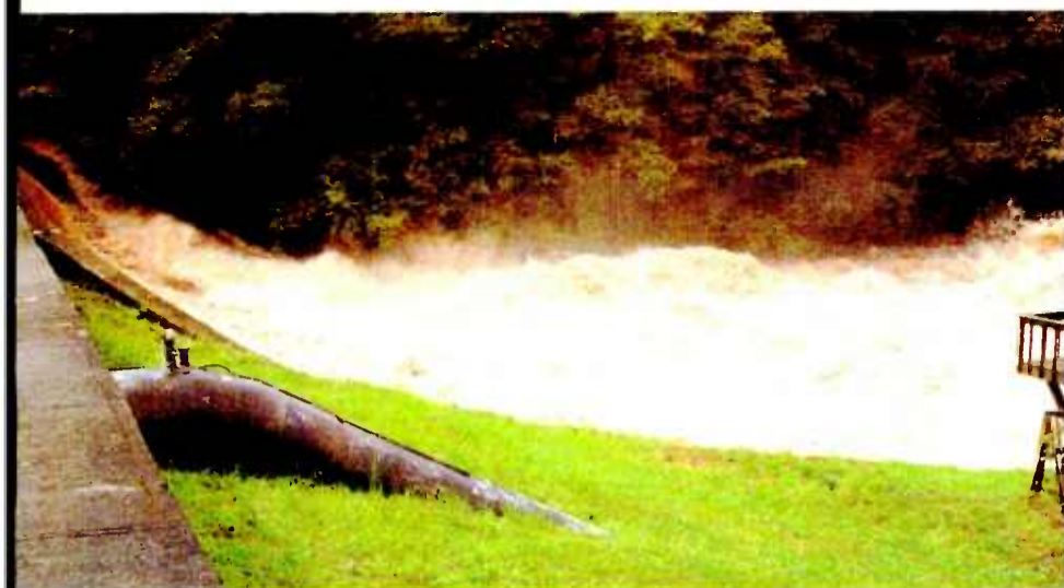
A 'penstock' at the base of the dam delivers water to the turbines in the powerhouse.
