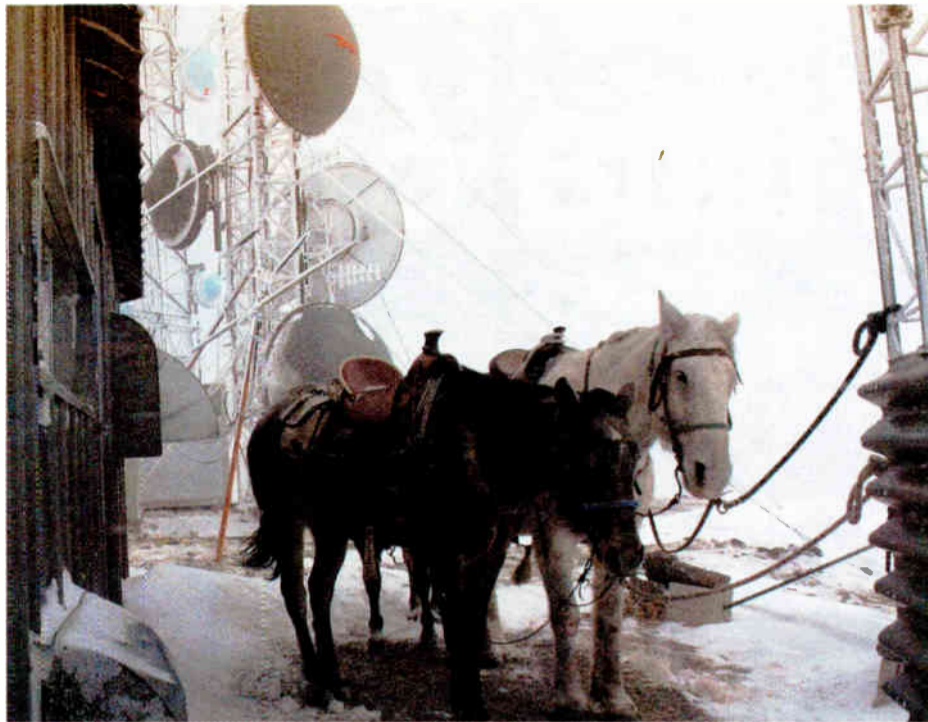
At the tower site.
