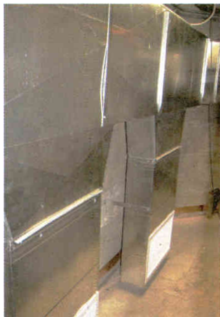
Fig. 2: Use a Digital Day Counter to keep tabs on when to change filters.
