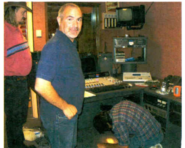
Crawford Denver Chief Engineer Ed Dulaney, left, and St. Louis CE Rick Sewell look on as Keith Peterson makes wiring connections to the KLTT Wheatstone Generation-5.
