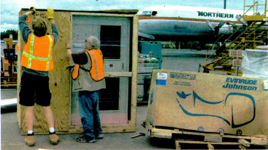
Service on the fly: Contract Engineer Bill Prendergast, left, and APBI DOE Chuck Lakaytis had to disassemble this transmitter on the tarmac at Anchorage Airport to make it fit in a DC-6.
