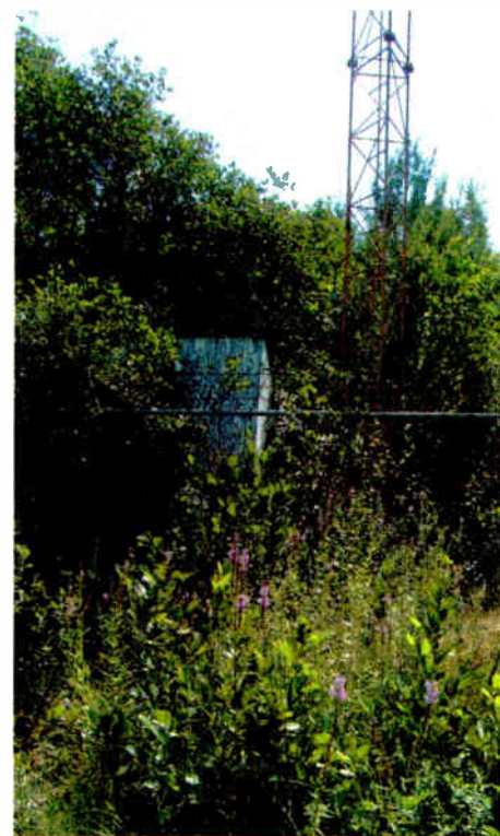
Fig. 2: Use winter months to schedule tree or landscape help. Keep your towers clear.
