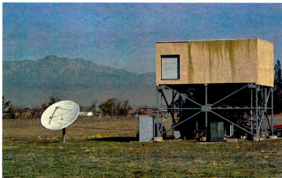
The transmitter site of KLAA(AM).
