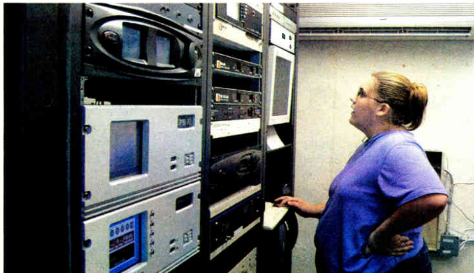
Timmons creates and saves an operations log using Burk's Autopilot 2 software. She handles routine weekly maintenance at the WGYS transmitter site in Frederick.
