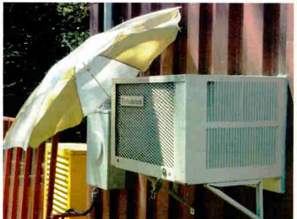
Fig. 2: The umbrella increases an air conditioner's efficiency.
