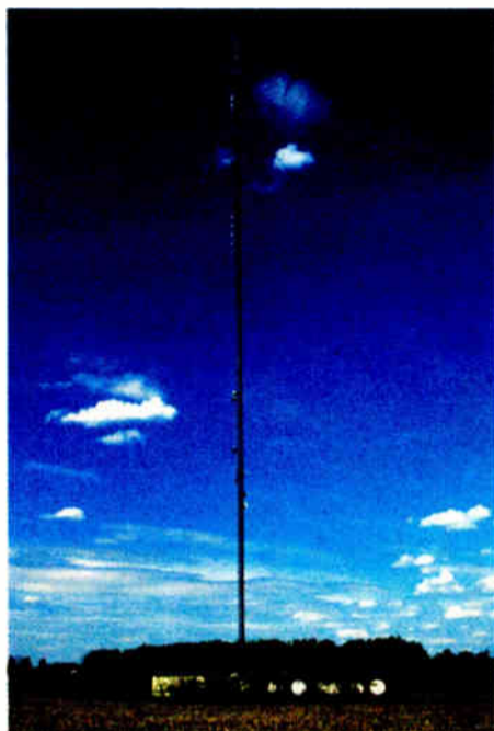
A Valmont 700-foot guyed tower in Mishawaka, Ind.
