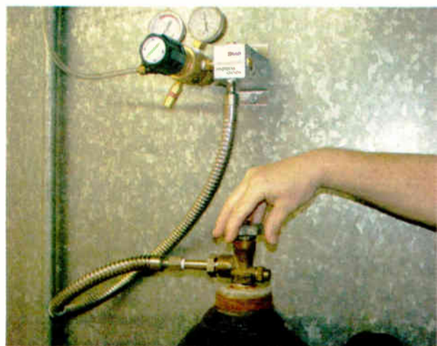
Fig. 1: This type of regulator mounts your gauge assembly to the wall.
