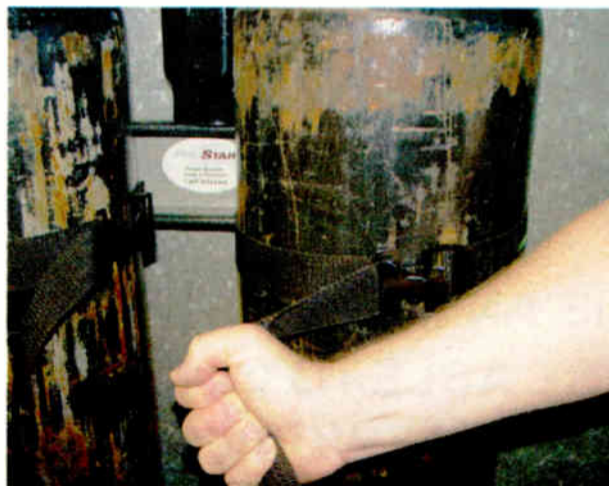
Fig. 2: Use a quick-release webbed belt to secure nitrogen tanks.
