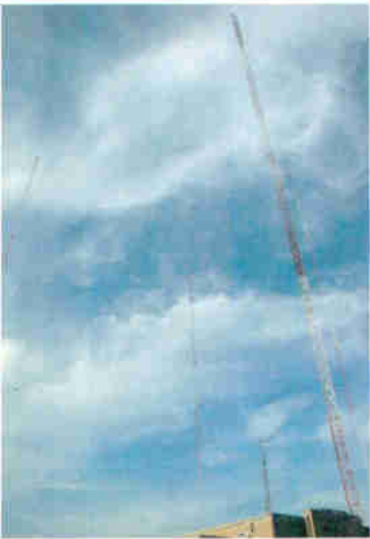
The venerable 1250 (former WEMP) transmitter towers.
