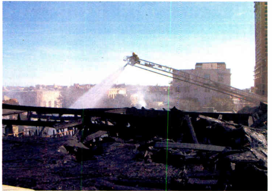
A view from KOOP's main studio during its initial damage assessment walk-through with the fire department. Firefighters are seen dousing hotspots.
