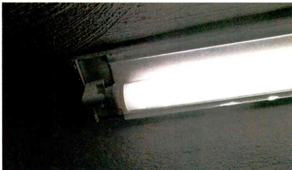
Fig. 1: A clear plastic sleeve protects florescent bulbs.
