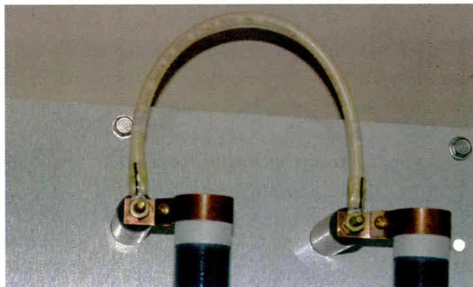
Fig. 2: Keep bleeder connections clean and tight.
