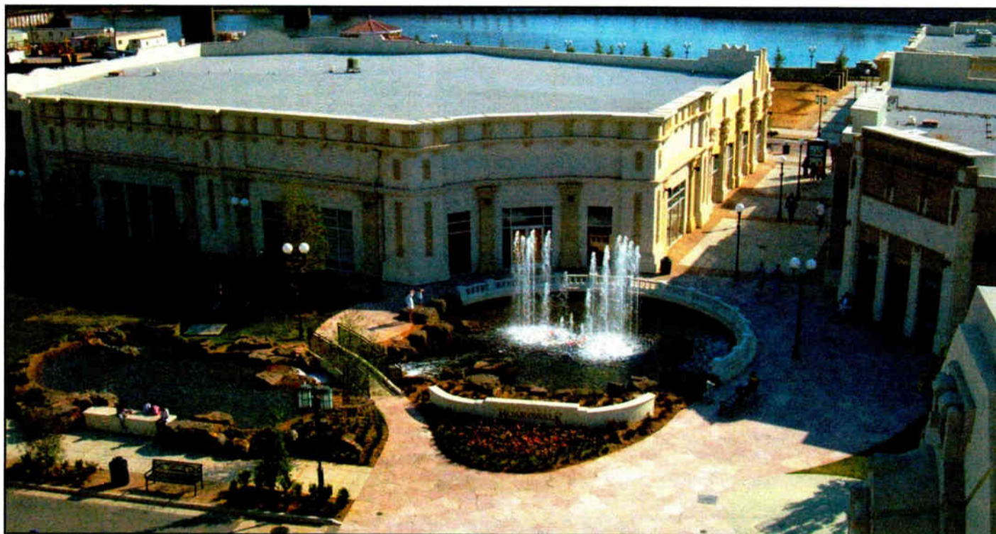
A view of the Louisiana Boardwalk.
