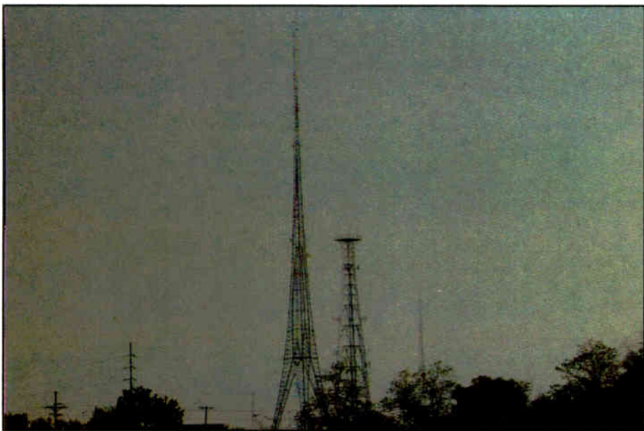
KVMA(FM) and KRMD(AM) operate from a self-supporting tower (left) three miles south of the new studios in Shreveport. Its design earned it the nickname, 'Eiffel Tower.'
