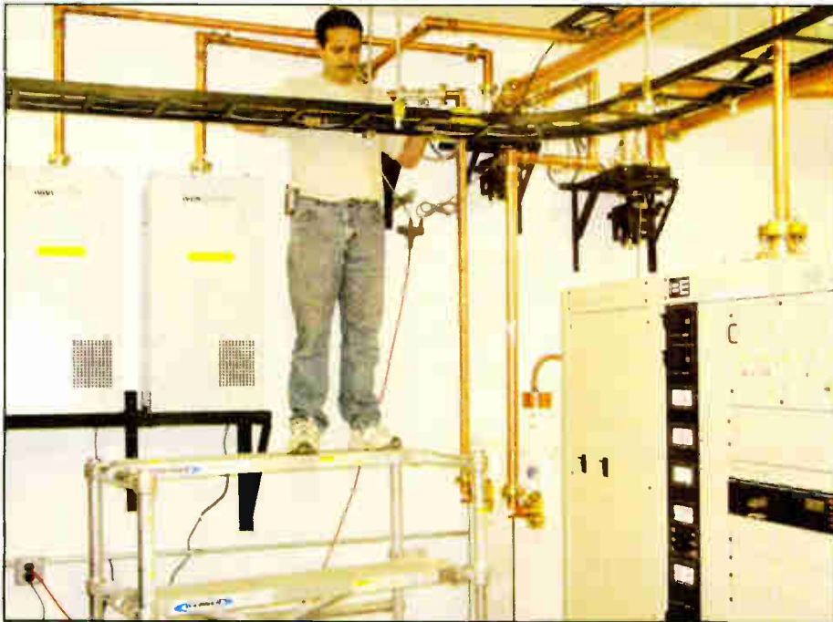
Fig. 1: A portable scaffold expedites transmitter site construction.
