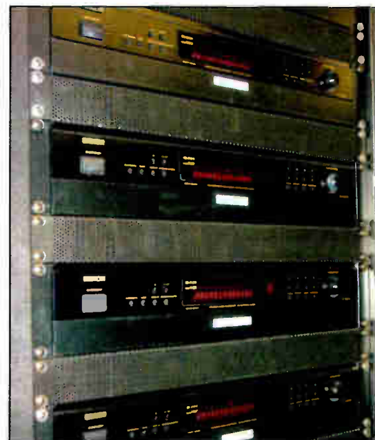
Fig. 3: Use perforated panels for rack ventilation.
